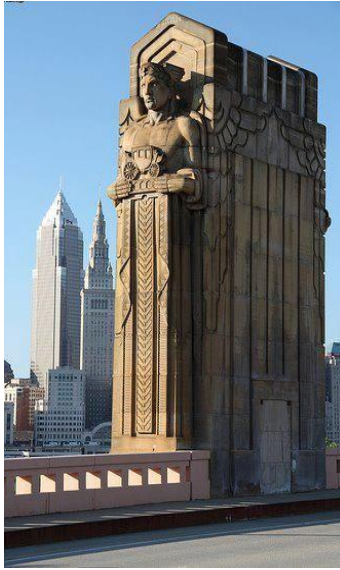
IMG 2.16 Hope Memorial Bridge 48 CLEVALAND, OHIO, USA
