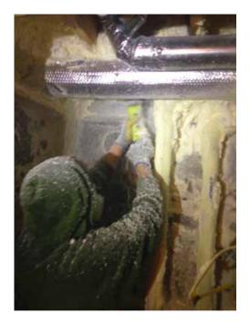
Figure 3.2 Trimming and removal of closed-cell foam using a powered brush tool. Source: Author's own elaboration
