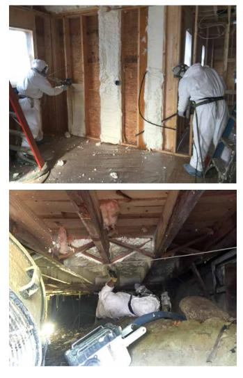
Figure 3.1 Spray foam insulation of (A) a new building (open-cell type) and B) the basement of an old house (also open-cell). The second worker in (A) is trimming the foam with a blade saw. Source: Author's own elaboration
